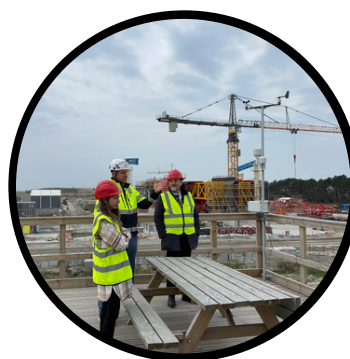
Danitacom's General Secretary Chiara Dell'Oro Nielsen during a visit to the construction site of Fermhen Belt
